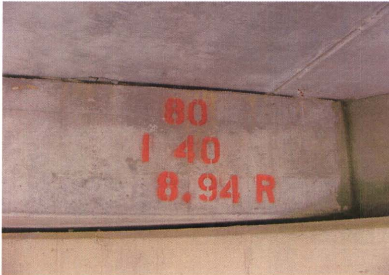
BRIDGE NO. AT ABUTMENT # 1
