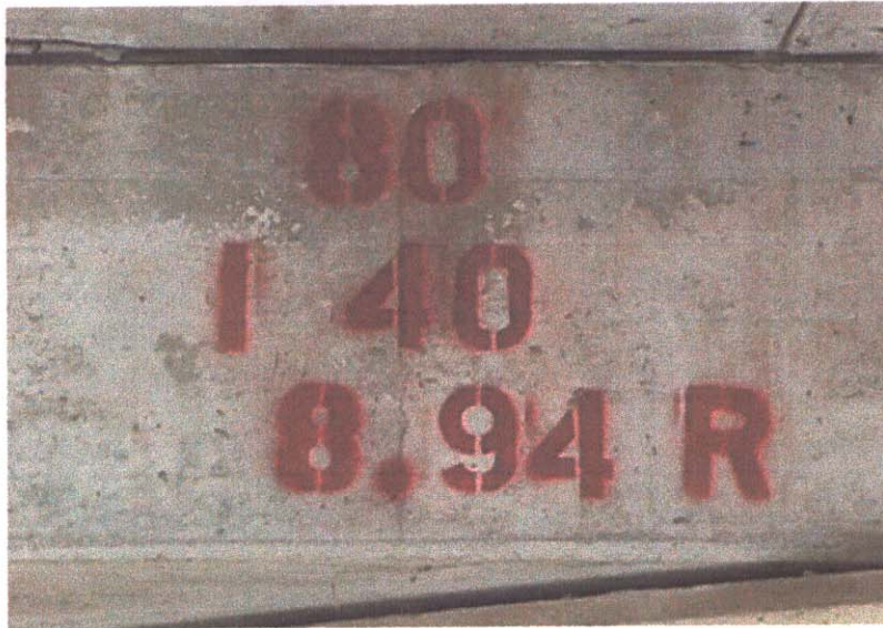
BRIDGE NO. AT ABUTMENT # 1
